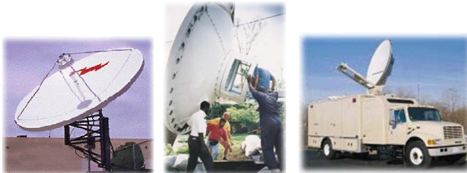
Figure 1 - Typical Earth Station Configurations
